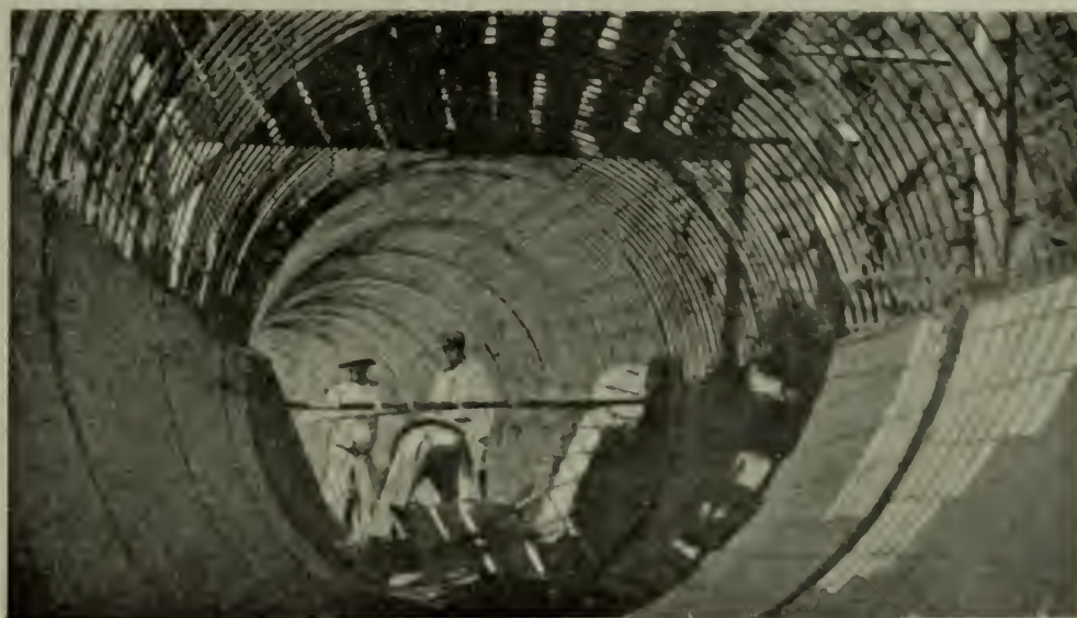
FIG. 9. CONCRETING INSIDE A CONDUIT OF 8 FT. DIAMETER.
